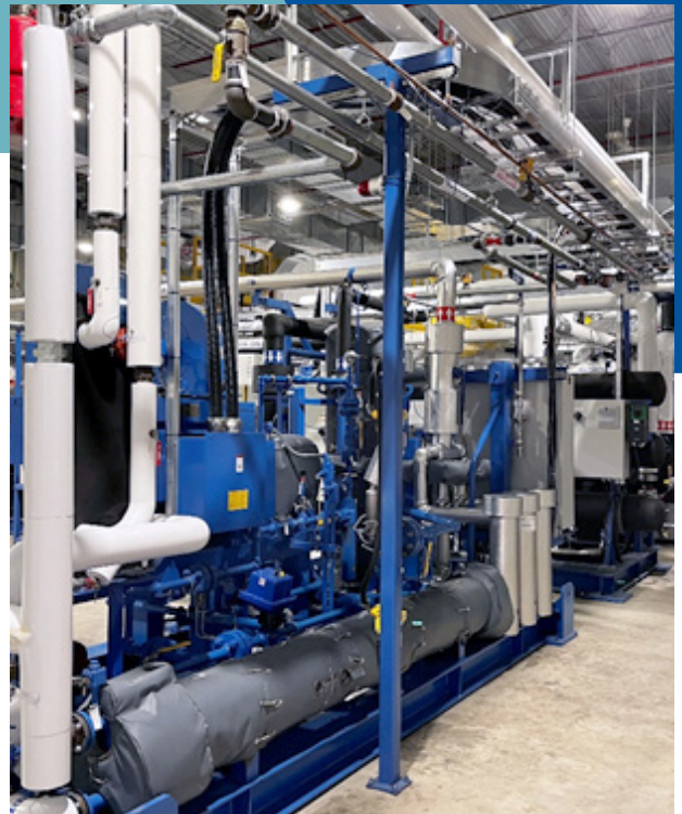
The Emerson CO 2 heat pump in operation at the Hydro Quebec Energy Technologies Laboratory in Shawinigan, Quebec produced 99.6 percent less Greenhouse Gas (GHG) emissions in testing.
